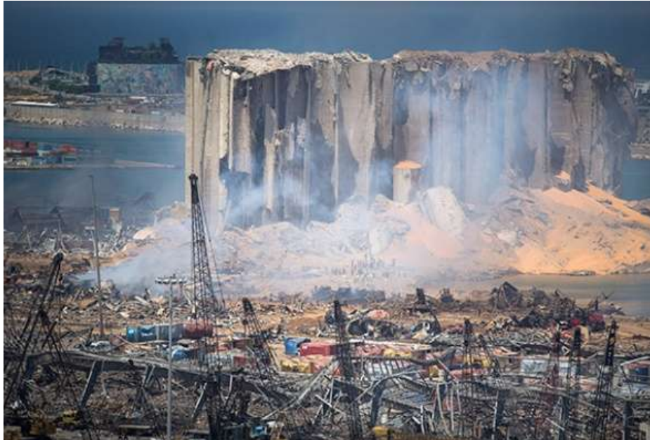
The blast rocked the Port of Beirut shaking buildings all over the city and causing massive casualties and damages.
