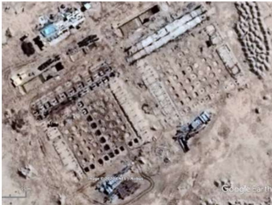
A Google Earth image taken showing buildings early in the construction process at the suspected nuclear facility.
